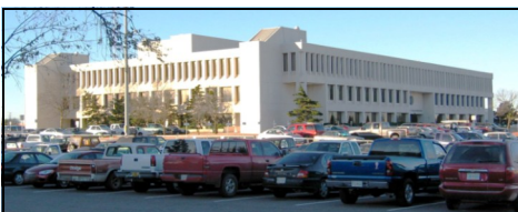
Department of Transportation Building Current Rating: 68 (E)
